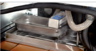
TAC Condensate Heater Pan/Bracket Kit Pictured without back screen.
